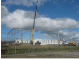
building has begun
