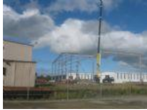
building has begun
